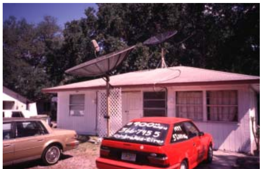
ANTI-PEDESTRIAN DEVICE: A LARGE RADAR DISH BLIGHTS ITS NEIGHBORHOOD.
