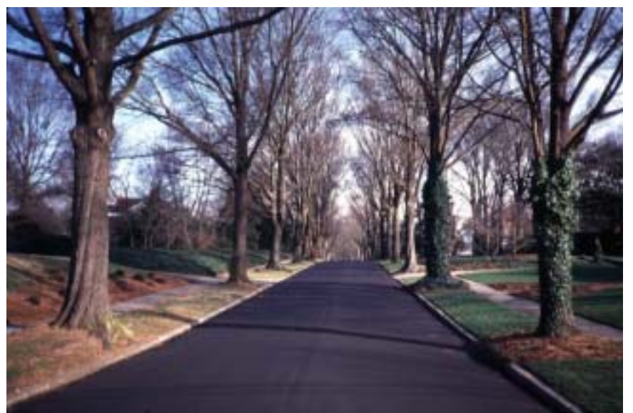
CHARLOTTE, NORTH CAROLINA: AN ASPHALT SURFACE, SIMPLE CONCRETE CURBS AND SIDEWALKS, AND ALIGNED TREES MAKE FOR AN IDEAL RESIDENTIAL STREET.
