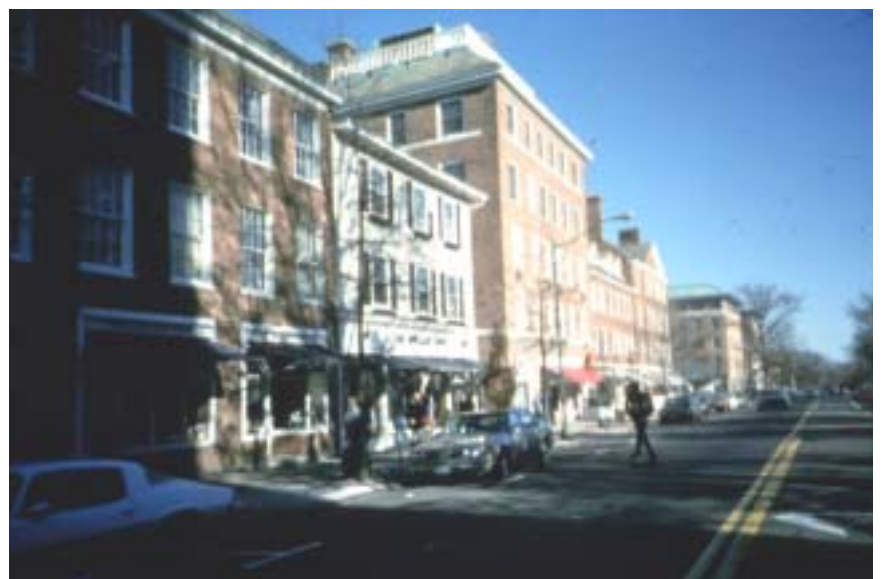
PRINCETON, NEW JERSEY: OFFICE SPACE (AND HOUSING) ABOVE RETAIL CREATES GREATER DEMAND FOR THE RETAIL AND GREATER CONVENIENCE FOR THE OFFICE.
