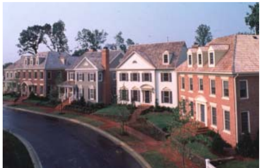
STREETS WITHOUT GARAGES: IN KENTLANDS, MARYLAND, REAR LANES ALLOW HOUSES ON 50'-WIDE LOTS TO LOOK LIKE MANSIONS.
