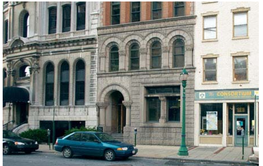
HANOVER SQUARE: OLDER BUILDINGS WITH CLEARLY DEFINED ENTRIES
