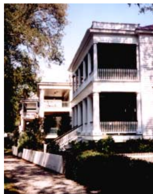
NEWPOINT, SOUTH CAROLINA: PORCHES ARE 10' DEEP, WHICH ALLOWS THEM TO BE TRULY USEFUL.
