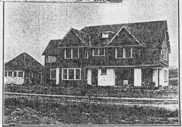
Residence of Judson W. Clark, Cor. Strathmore Drive and Wellesley Road. It will soon be ready for occupancy. Hollow tile and frame construction, Ward W. Ward, Architect
