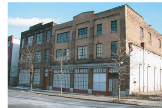
Many older structures contain interesting architecture. Source: Author, 2006
