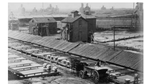
Syracuse Salt Sheds and Solar Evaporation, 18... Source: "Erie Canal Museum: Photos from the Collection" Erie Canal Museum. Syracuse, NY. 1989.
