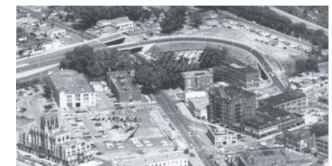
Construction of West Street Arterial at West Genesee Street Source: Onondaga Historical Association Museum, Archives Division. Folder: Block 66. Syracuse, NY
