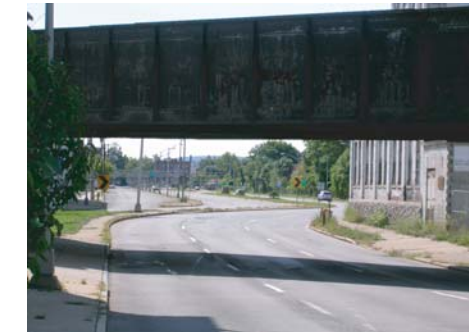
South West Street, Looking South at DLW Rail Bridge. Source: Author, 2005.
