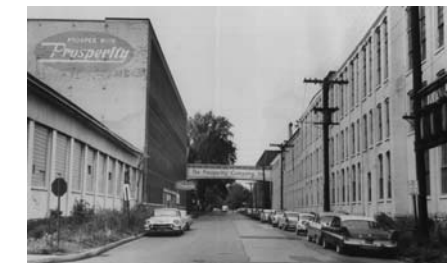
Industrial Fabric. Looking West at South West Street and Marcellus Street, circa 1950s. Source: Onondaga Historical Association Museum, Archives Division. Block 242 Folder: Photography Syracuse, NY.
