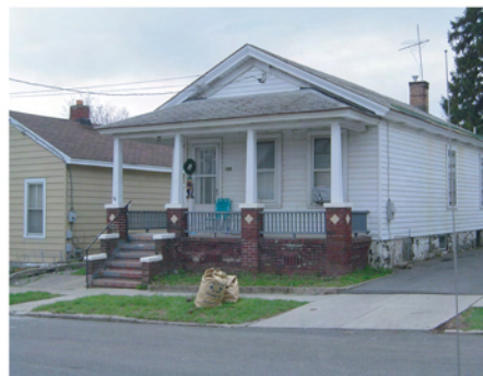
Existing, Worker House on Peters Street
