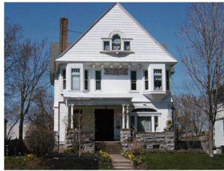
Existing, Single-Family House on Park Avenue
