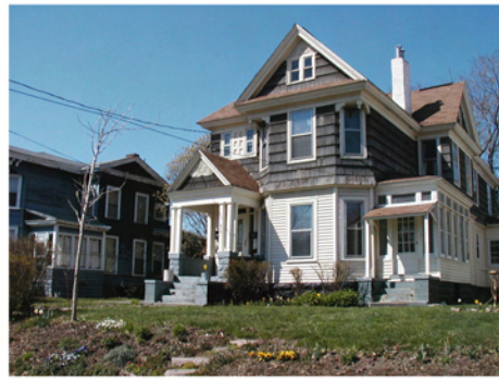
Existing, Two-Family House on Park Avenue
