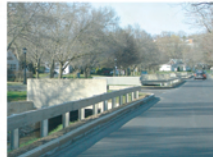
Existing, Meadowbrook Drive
