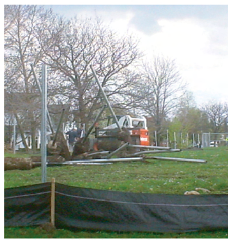
Fence replacement in Salem Hyde neighborhood playground.
