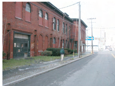
Existing, 500 Townsend Street, Water Street
