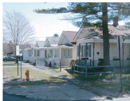
Existing, Streetscape on Carbon Street
