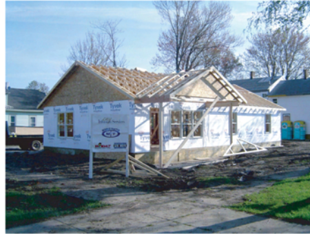
New construction on Southwest neighborhood.
