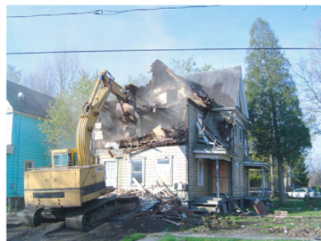
Building demolition on Westside.
