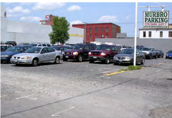
Inappropriate use of material and lack of surface markings for parking bays and drive lanes.
