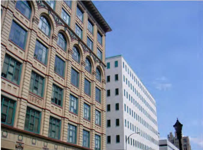
Inappropriate transition in bulk, materials, and scale that does not reflect traditional urban patterns of adjacent buildings.
