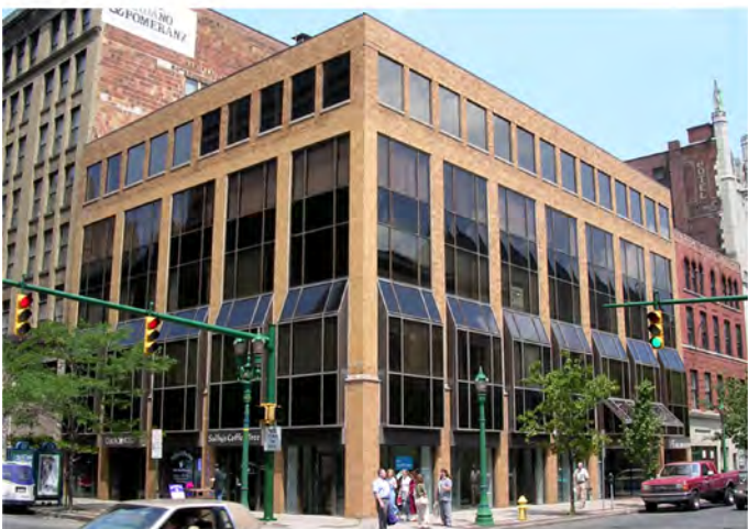
Inappropriate window character that is inconsistent with traditional Downtown buildings.
