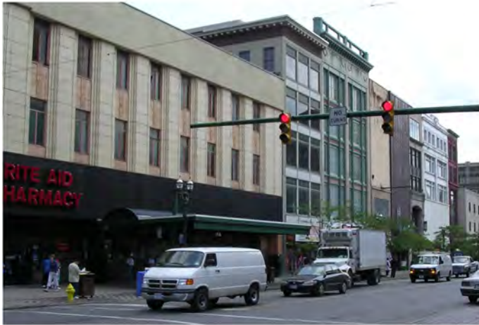
Inappropriate storefront articulation that does not provide traditional physical and visual links between public space and building interior.
