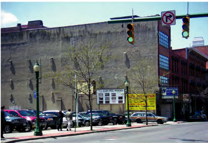
Inappropriate informational and directional signage which creates visual clutter.
