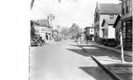
15th Ward, c1950. The residential character of this section of Downtown was lost in demolition under the Federal Urban Renewal Program.
