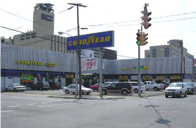
Inappropriate signage that does not fit the scale and character of the building.
