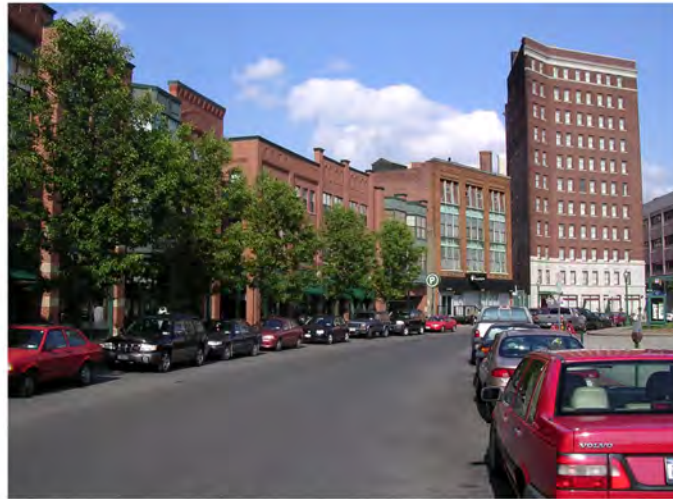
Compatible buildings in terms of bulk, materials, and scale reinforce traditional urban density and form.
