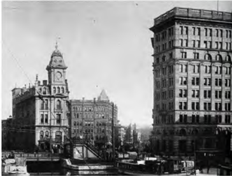
East Genesee Street corridor: view to Fayette Park.
