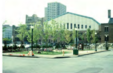
Park and parking lot prior to construction of Center Arroyo.
