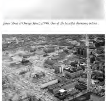
The 15th District, c1965, after demolition.
