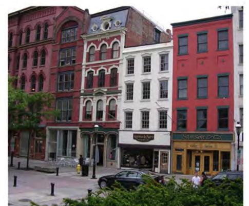
First floor retail in Hanover Square.
