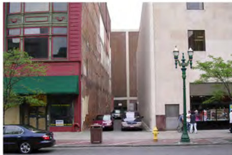
Demolished building on South Salina Street.
