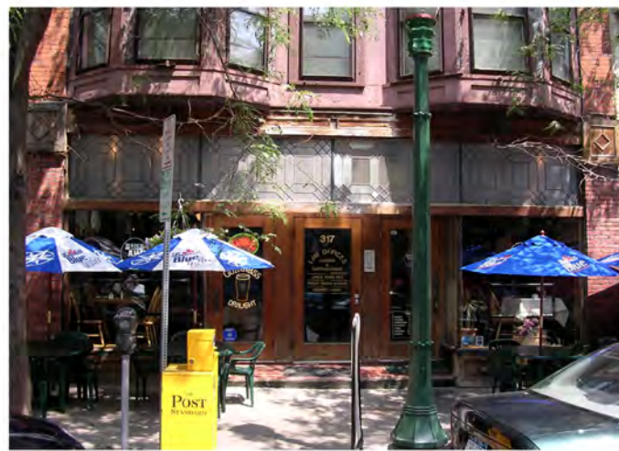
Appropriate facade treatments enhance the street corridor.
