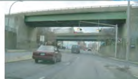
Existing conditions, North Salina Street.
