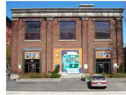
The Former Trolley Barn on North Townsend Street
