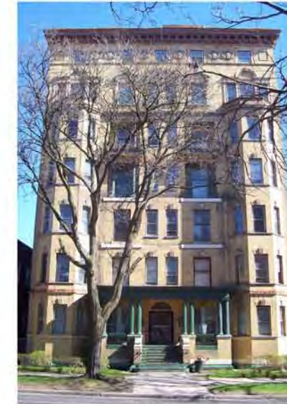
Kasson Apartments - 622 James Street
