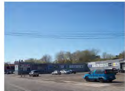
Existing, view looking north-west from Burnet Avenue toward Ra-Lin
