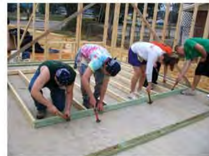
Volunteer community building project
