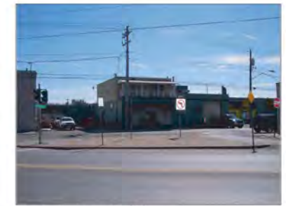
Existing, looking at Lodi Street
