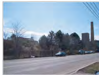
Existing, ROW along Burnet Avenue
